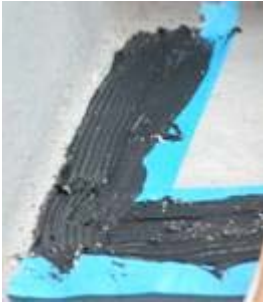
Margin taped and Adhesive applied.
